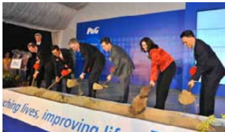
January 27, 2011: Procter & Gamble executives break ground on its Singapore Innovation Center, the company’s global state-of-the-art research facility in Singapore’s Biopolis, which is slated to open in 2013.
